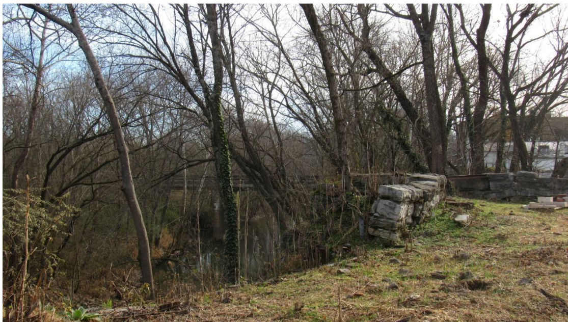
Civil War era bridge (right) with current bridge in the background
